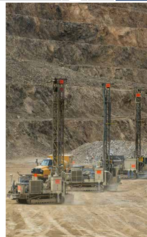
Drilling blast holes at Fort Knox
